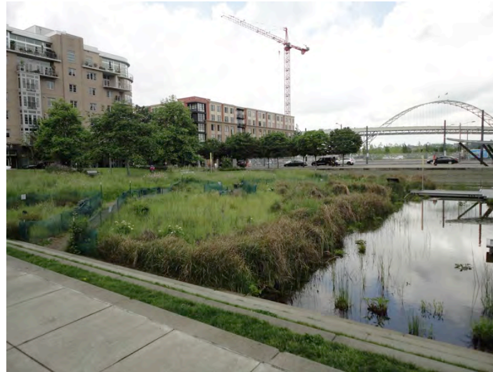
TANNER SPRINGS PARK, PORTLAND, OREGON STORMWATER MANAGEMENT SYSTEM
