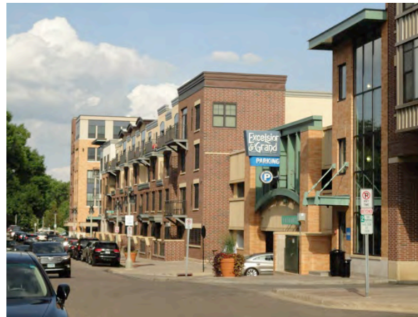
ENTRANCE TO PARKING STRUCTURE IN THE CENTER OF THE BLOCK
