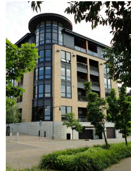
ENTRANCE TO UNDERGROUND PARKING
